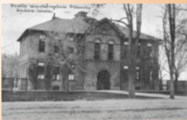
SOUTH WASHINGTON SCHOOL - 3279 Washington Blvd, built 1904. Demolished in 1990s, now a park.
