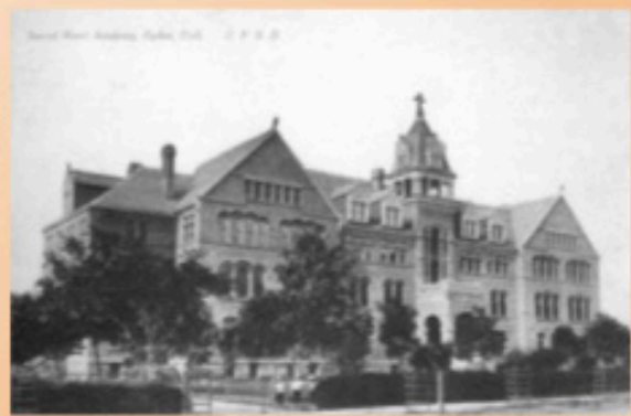
SACRED HEART ACADEMY- 25th Street between Jackson/Quincy Built in 1902 and demolished 1950s
